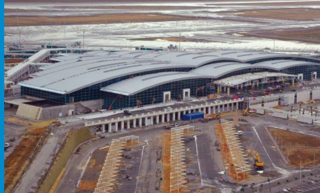
Bodrum airport - Turkey
