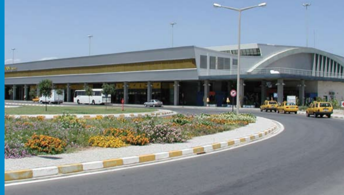
Tbilisi roof renewal - Georgia - International Airport
